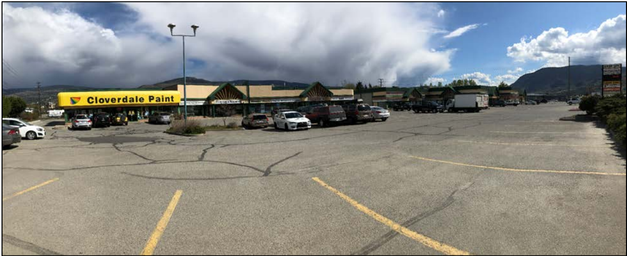
Figure 5 – Looking east towards strip mall buildings on subject property
